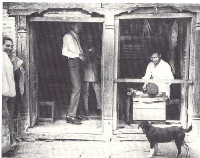
Fig. 1. A carpenter's shop in the city of Patan
